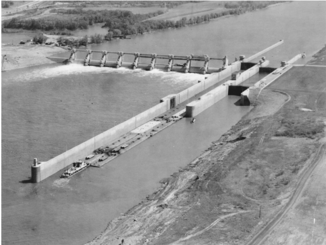
Figure 2-1. Parallel locks with gravity walls. Willow Island Locks, Ohio River, with design lift = 20 ft
