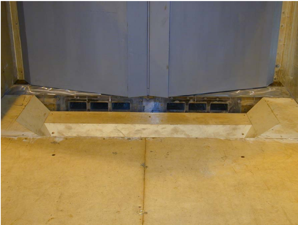
Figure I-4. View of through-the-sill intake for J. T. Myers lock extension
