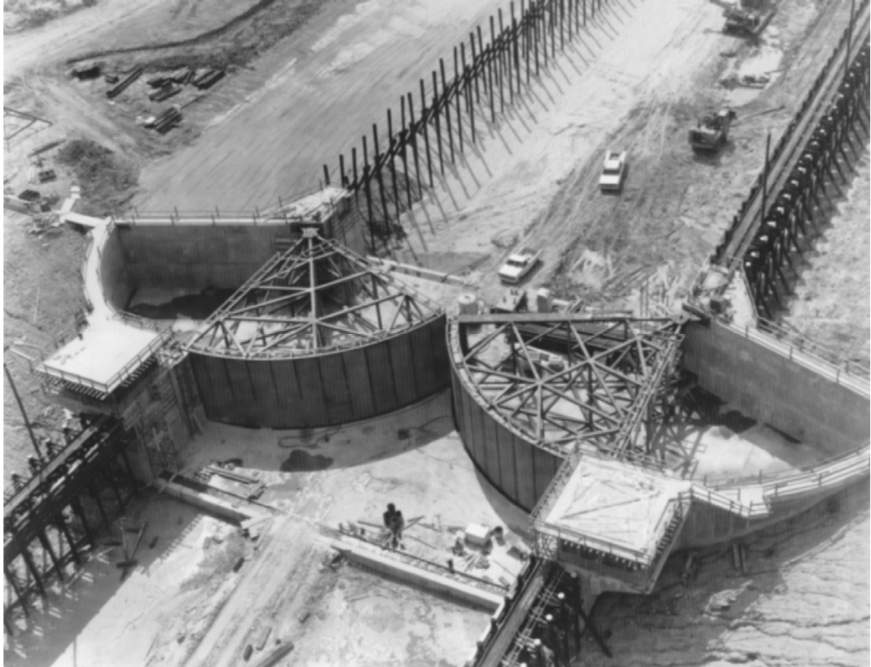
Figure 2-6. Earth embankment with concrete gate bays and sector gates. Vermilion Lock, Gulf Intracoastal Waterway, with design lift = 3 ft (under construction, 1984)
