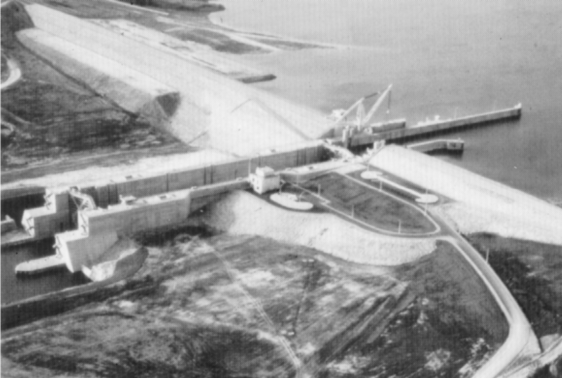
Figure 2-4. Lock with thin walls. Bay Springs Lock, Tennessee-Tombigbee Waterway, with maximum design lift = 92 ft
