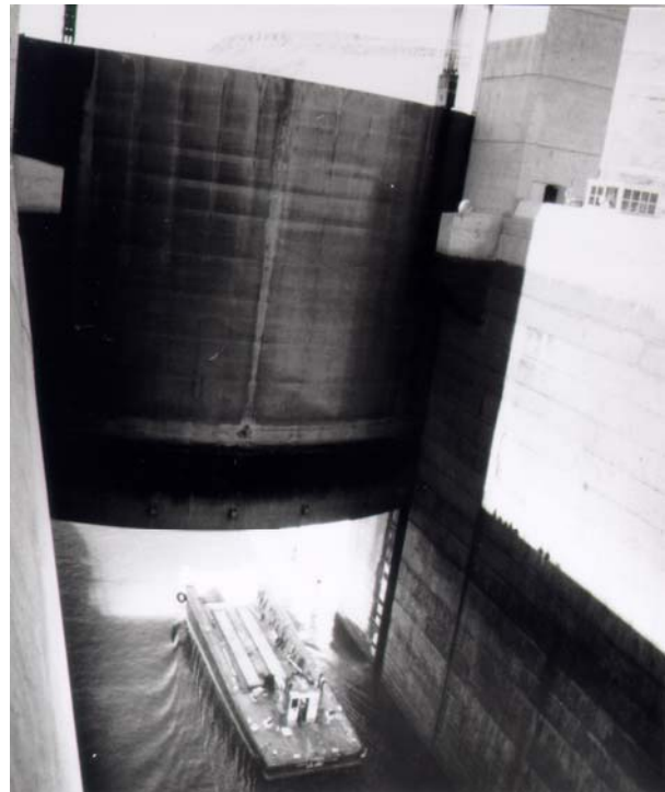
Figure B-4. Overhead vertical-lift gate
